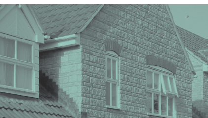
Type G cavitytrays with attached lead flashings provide protection to the front horizontal intersection. Note the Type X trays used above the sloping abutment terminate with an external angle. This provides a protective link with the Type G trays.
