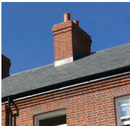
Chimney stack showing lead work. Also shown at lower level is brickwork corbel where airflow to the roof space is provided via a discreet corbel ventilator – see Ventilation section for details
