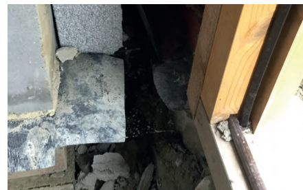
Site form barriers amalgamating with structural openings are commonly poorly executed, of questionable gas resistance and permit damp permeation.
