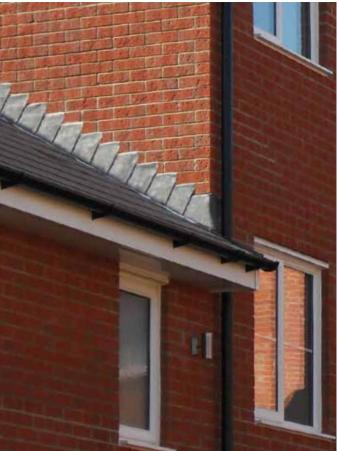
Type CRSS Continuous Running Soaker Strip at slate/wall junction with Type X Cavitray flashings dressing over CRSS upstand
