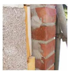
Full fill modular insulation is commonly out of alianment or finished too far back from the reveal face. Consequently there are gaps (hidden from view) between the insulation and a conventional cavity closer
