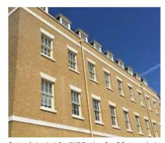
Cavity walls closed with Type FWC Cavicloser. Type C Cavitrays at lintel level, Discreet Caviweeps located in brickwork beyond surround feature
