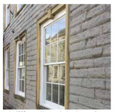
Insulated DPC is not visible in typical sash window re-installation
