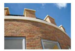
The conventional cavity parapet is normally terminated with copings, under which a DPC is bedded. The width of the DPC is required to be sufficient to slightly overhang the width of the parapet masonry. Support of the DPC is required where it crosses the cavity. The Type J Support and Closer is designed for such purposes.
