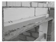
Uniformity and consistency can be difficult to achieve using soft roll DPC but with a preformed Type C Cavitray the angle and dimensions can be specified and maintained.
