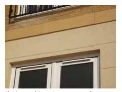
When closing reveals the opportunity exists to maximise thermal retention and consistent protection as the dpc is preformed and not susceptible to distortion or misplacement.
